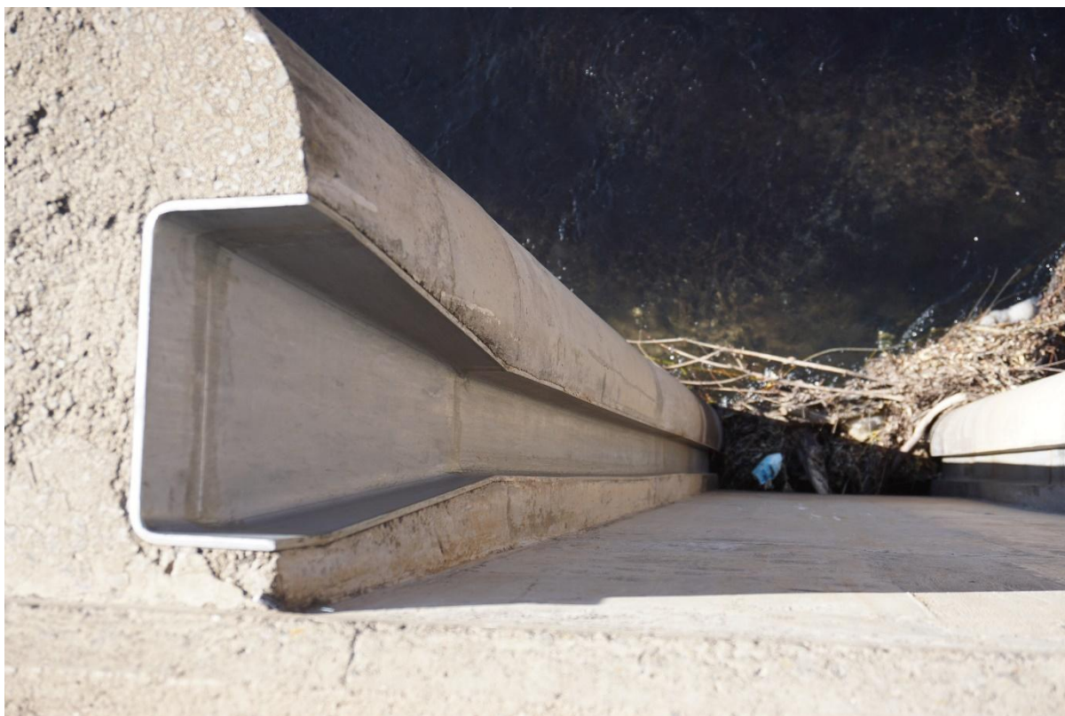
Figure 18. The screen guide channels as viewed from the top of the roof slab. The guides taper at the top.
