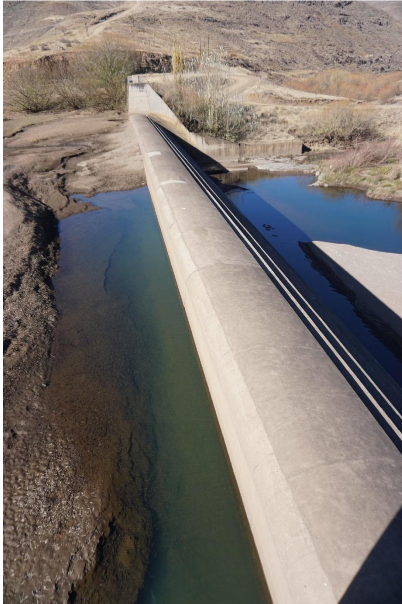
Figure 19. The ogee weir as viewed from the roof slab of the intake structure
