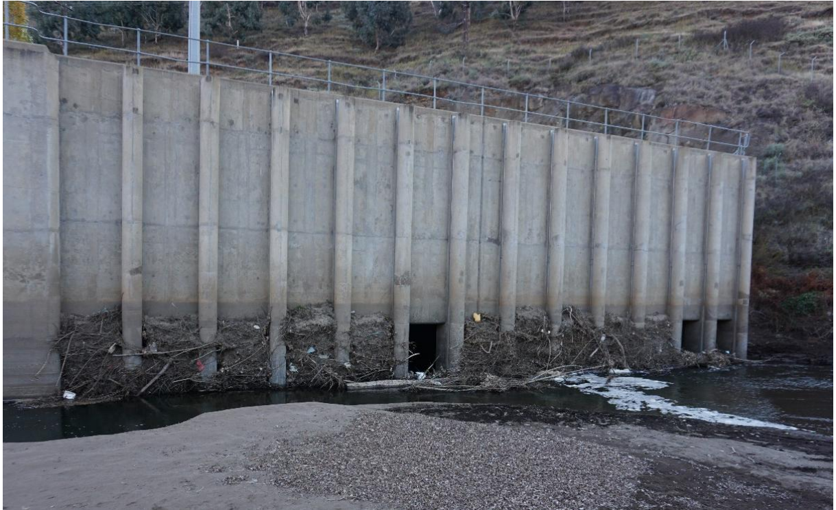
Figure 3. Blinding of the screens at Matsoku Weir (7 June 2022)
