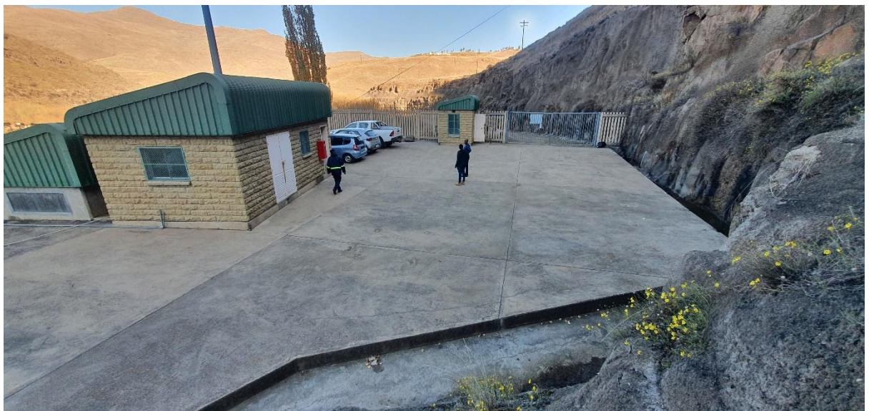
Figure 10. Entrance and access to the roof slab of the intake structure as viewed from the right bank. The roof slab is only accessible through a gate next to a guard house which is visible in the top right of the photo. The building provides access into the intake structure.
