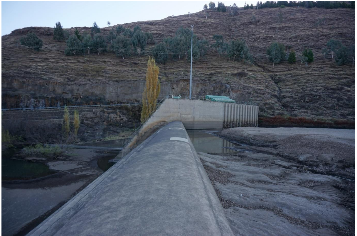
Figure 9. The Matsoku weir and divergence tunnel as viewed from the weir. The intake structure sits on the right bank of the Matsoku river. Water either enters the intake structure to flow to the Katse Dam or it spills over the weir.
