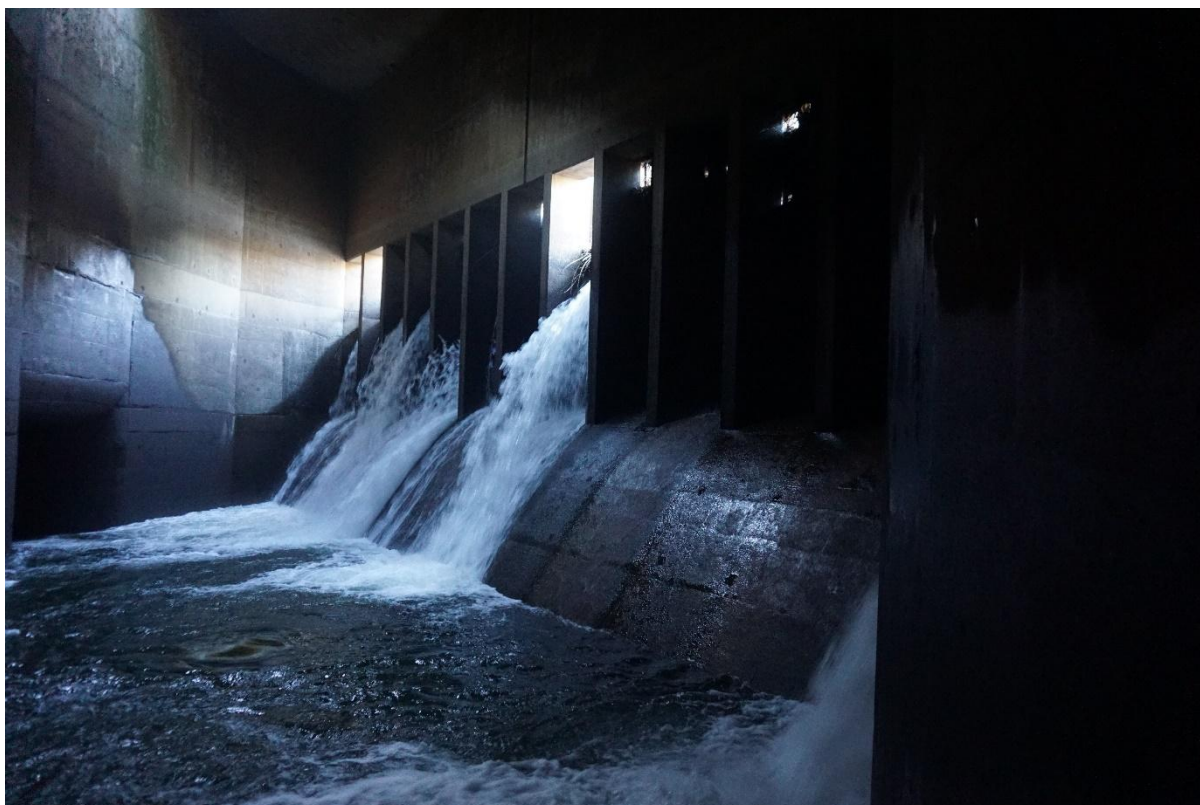
Figure 14. Inside the intake structure. The divergent tunnel is on the left. On the right are the thirteen screens. Some screens are completely blinded.
