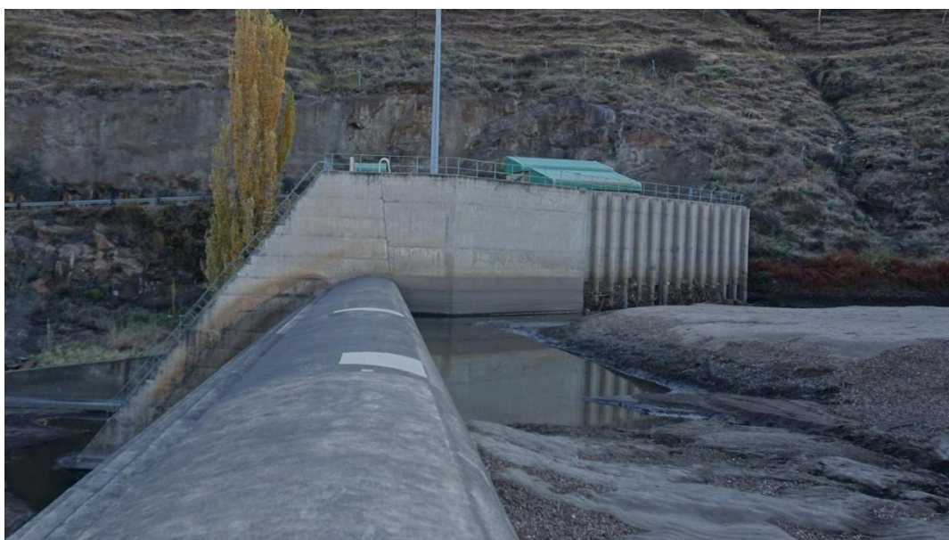
Figure 2. Matsoku Weir and Tunnel Intake Structure (7 June 2022)
