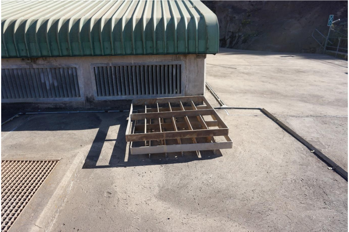
Figure 16. Two bar screen panels removed from the intake structure
